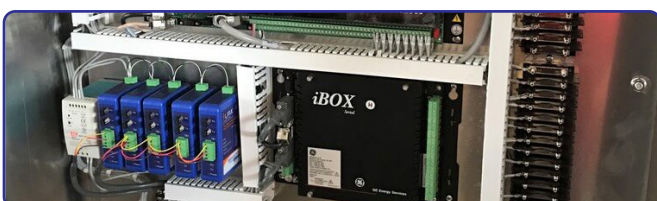
SCADA cabinet - endpoint state
